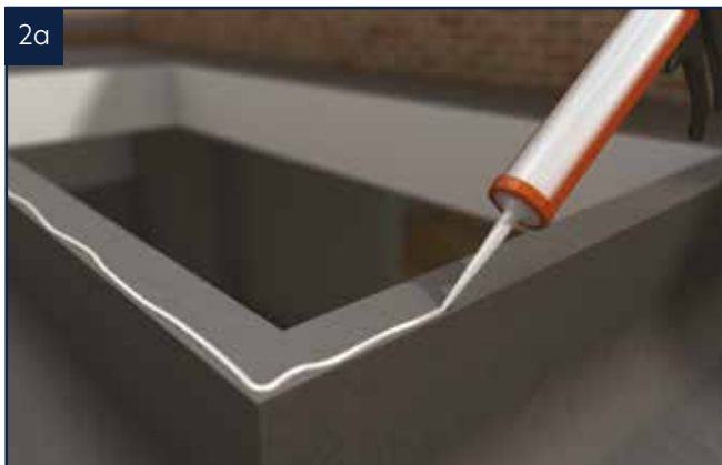
2a Apply a continuous bead of sealant to the outer edge of the upstand.
