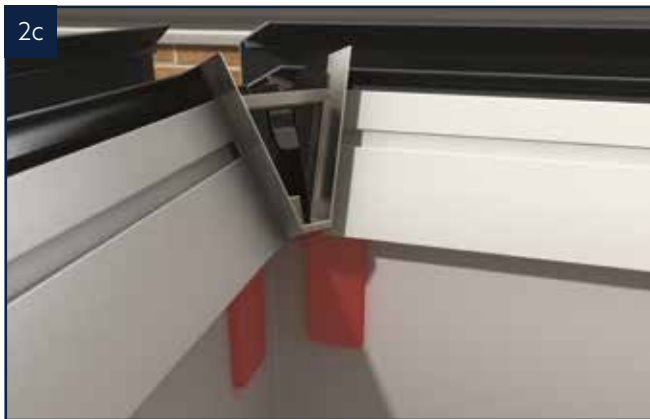
2c Ensure corners are tightly held against the aluminium. The corner connector assembly may need plastic packers behind if the upstand is not square or exact size.
