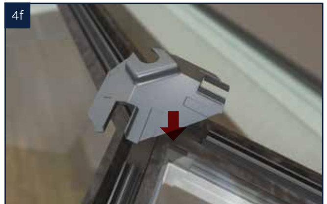
4f Position the ridge end seal in place ensuring it is central to the hip bars and ridge.
