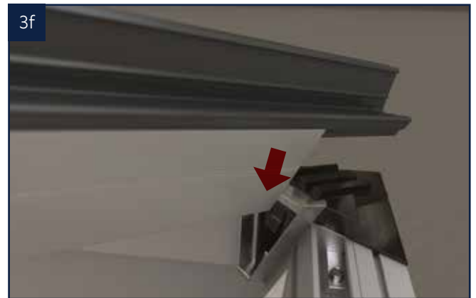
Ensure all the hips line up with the ringbeam corners. With a downward motion click the hips into place. Check all hips are locked into place at all four corners by applying an upward force on the hip.
