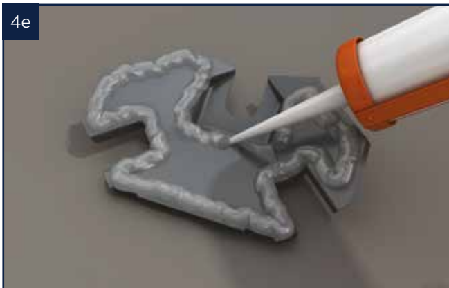
4e Apply sealant to the underside of the ridge end seal.
